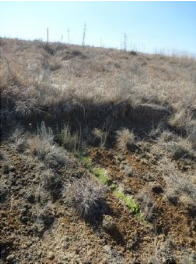
Figure 22 Road cutting with exposed flow (outside of a wetland area) at the end of July 2013
